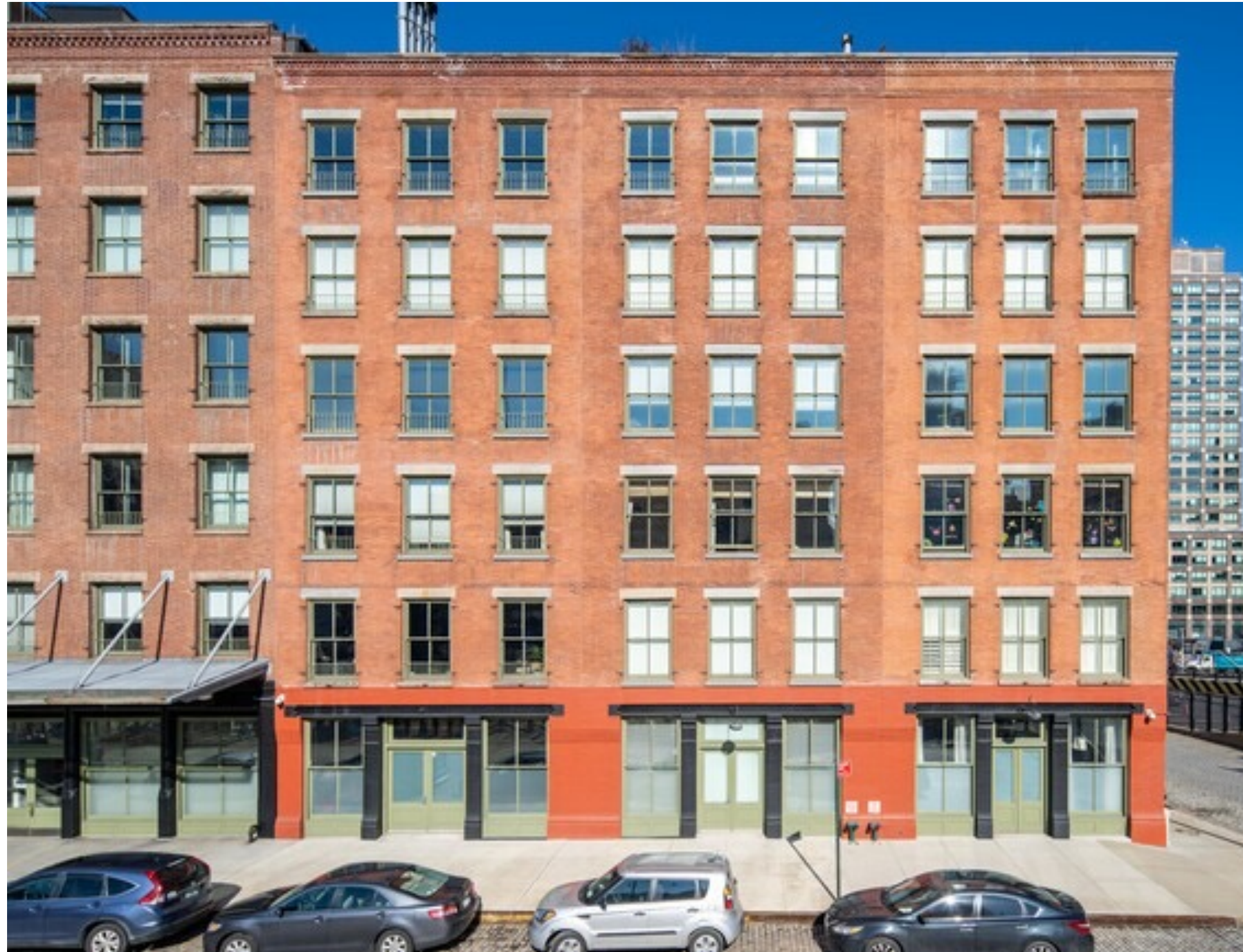
Cobblestone Lofts, Tribeca, New York City
