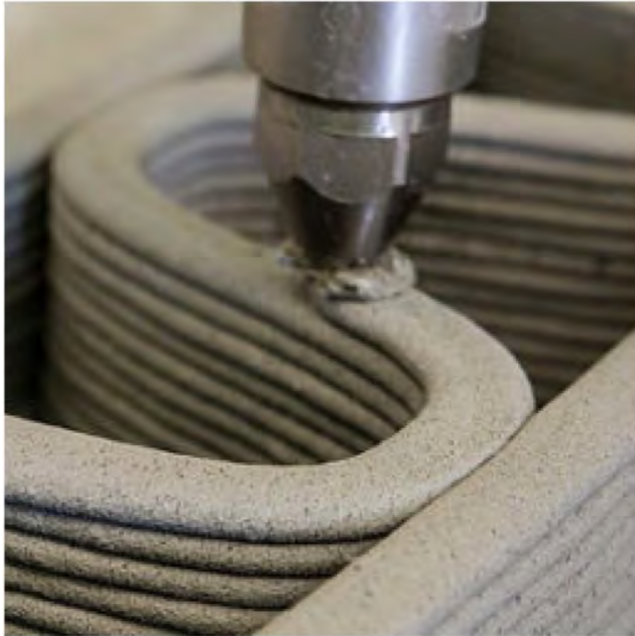
Manchester Metropolitan University - Concrete 3D Printing
